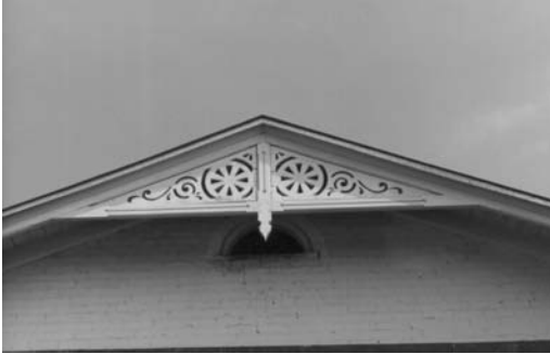
This scroll cut bargeboard decorates the gable end of this roof.
