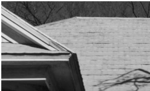
Pressed metal shingles are a common roofing material.
