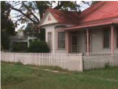
Wood picket fences should be restored.
