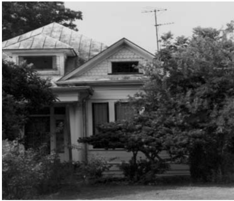
This roof form has a combination of hip, gable and dormer which is common to the neighborhood.
