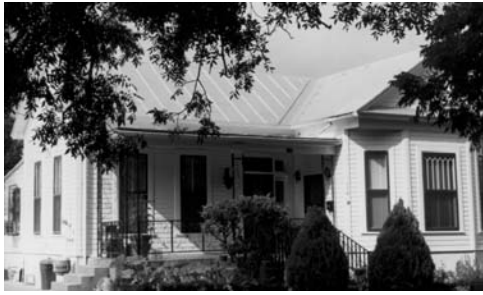
This house has fabricated metal porch columns and railings.
