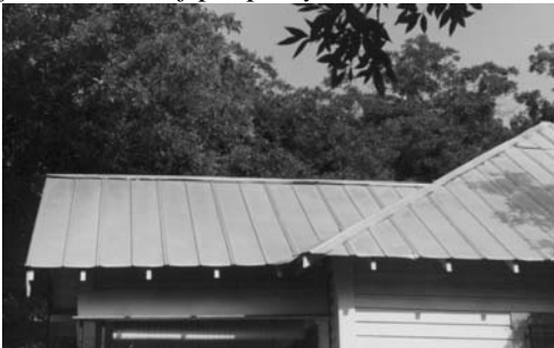
“V-crimp” metal roofing is an affordable alternative to composition shingle or a new standing seam roof.
