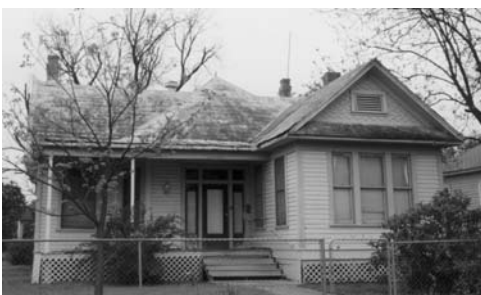
Lattice skirts allow for ventilation.
