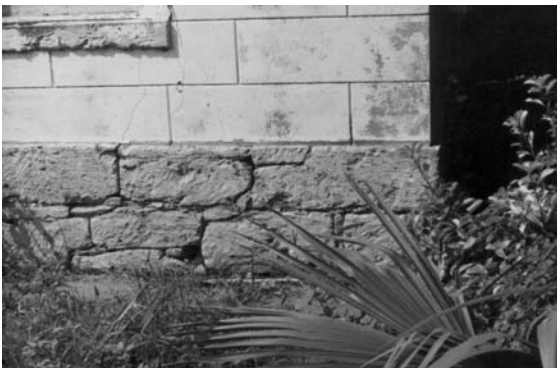
Repoint deteriorated masonry.
