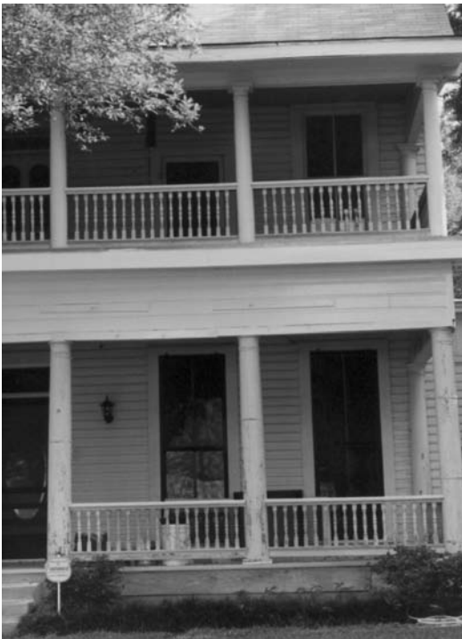
Retain and repair turned wood railings, columns and porch deck.
