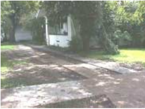
A concrete tire path driveway is a good alternative to solid paving.
