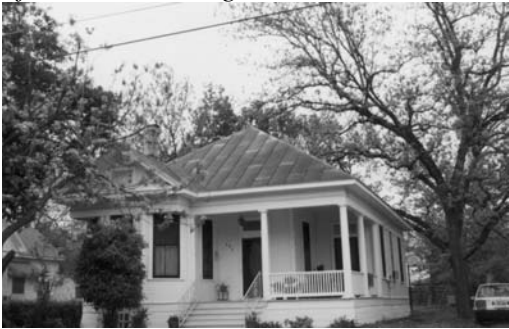
Standing seam metal roofs are common to the neighborhood and last for decades if properly maintained.
