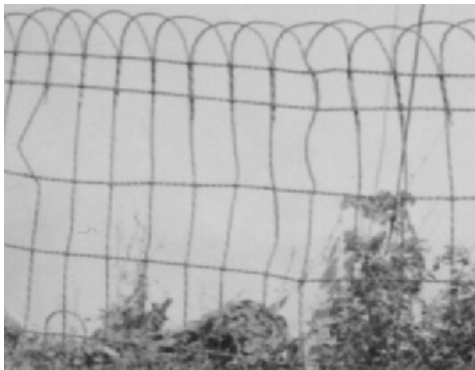
Garden loop wire fence is an appropriate alternative to non-historic chain link fencing.
