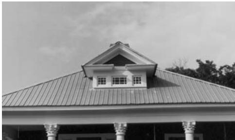
Capitals sit on top of columns and support the roof. The dormer projects above the roof the metal roof.
