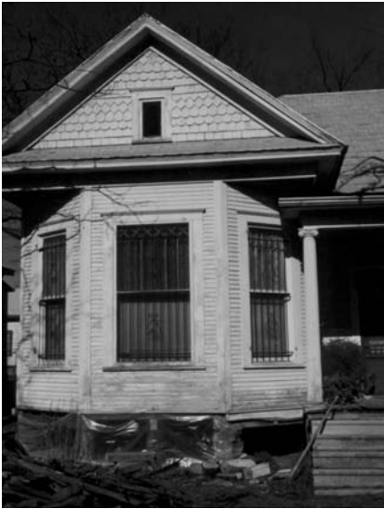
Cedar post foundations are common to wood frame structures.
