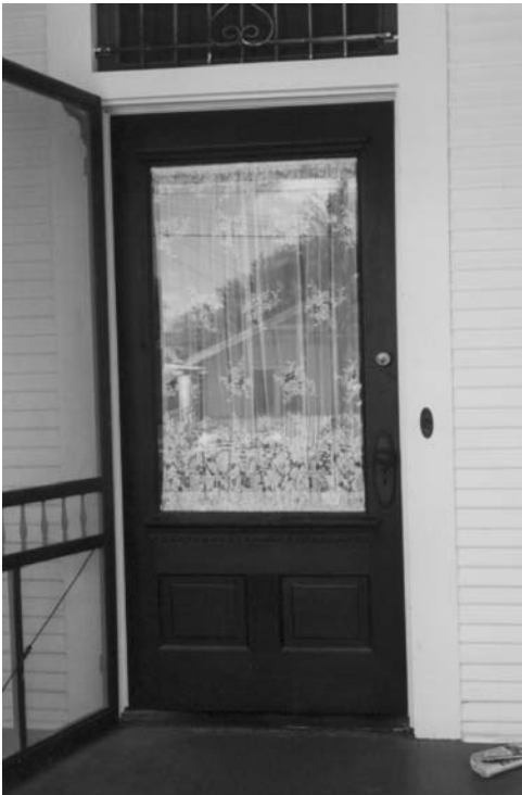
This is a typical historic front door with the upper glass panel, wood screen door and transom.
