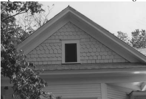
Boxed eaves, or overhang, are a typical detail in the neighborhood.
