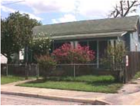
Porches frequently span the full front façade.
