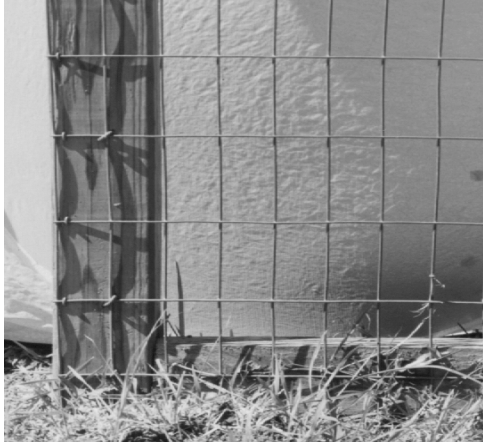
Welded wire fence called “hog wire” is an appropriate alternative to chain link.
