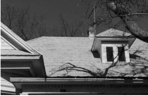
This house is covered in pressed metal “fish-scale” shingles.
