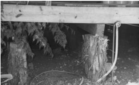
Pier and beam construction can be repaired with new wood members.
