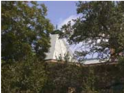
Many of the roofs are covered in standing seam metal.
