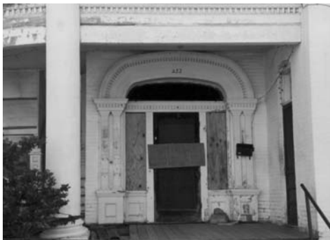
Transom and side lights are common at entry doors.
