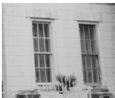
This 6 over 6 true divided light sash is important to the period of the house.
