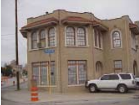
Fire Station No. 7 located at S. Alamo St. and Durango Blvd.
