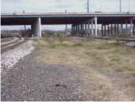
Existing conditions along Union Pacific Railroad
