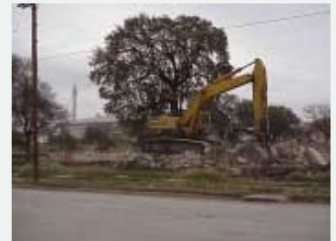
Demolition at the former Victoria Courts site
