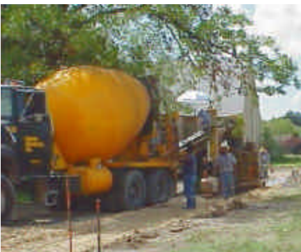
Construction crew at work in the planning area
