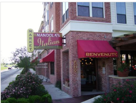
Attached signs are more appropriate than pole signs for higher density, pedestrian-oriented environments.
