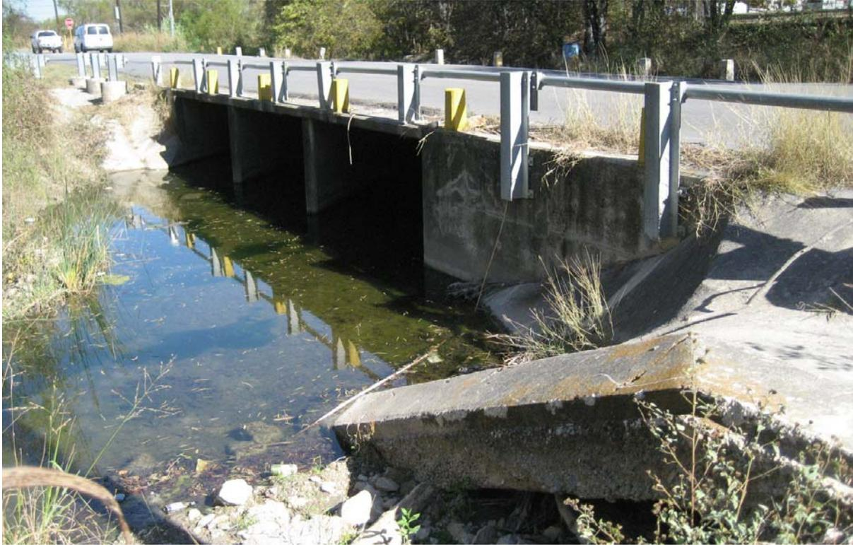
**Figure 6.** Box culvert bridge over Beitel Creek, looking northeast.
