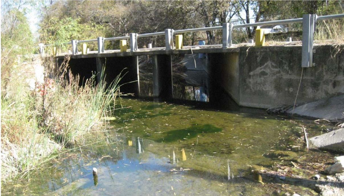
**Figure 5.** Box culvert bridge over Beitel Creek, looking east.
