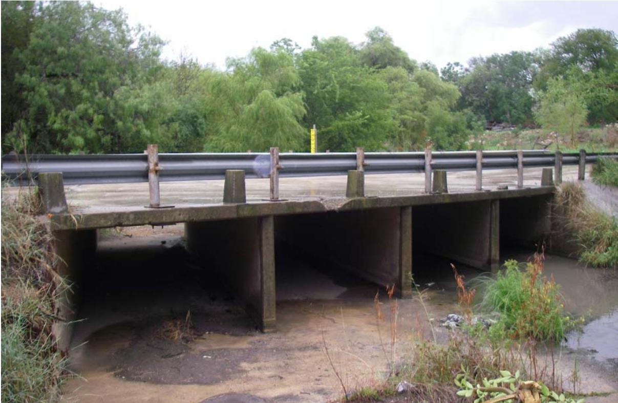
**Figure 6.** Box culvert bridge over Rosillo Creek, looking north.
